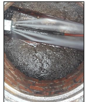
Emptying of blocked sewer manhole with venturi pump to remove foreign materials from sewer manhole
