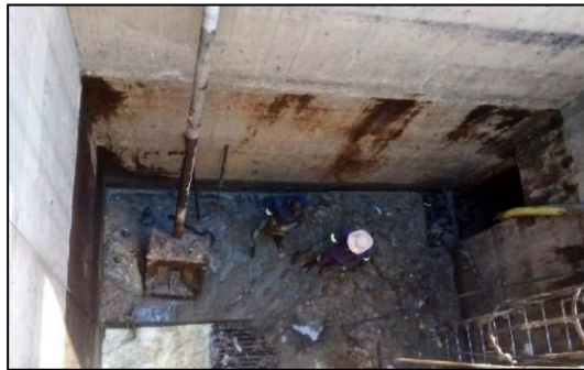
Silt and sludge being removed from sewer pump stations and large septic tanks.
