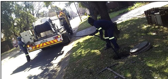
Emptying of blocked sewer manhole with venturi pump to remove foreign materials from sewer manhole
