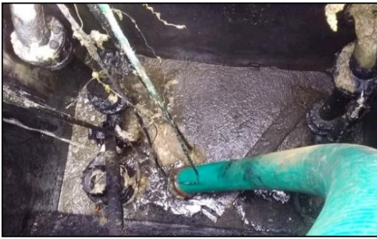
Silt and sludge being removed from sewer pump stations and large septic tanks.
